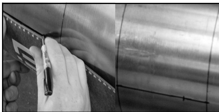
Figure 24: Marking the 9 o'Clock Position
