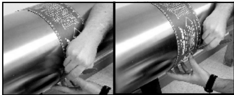
Figure 22: Marking Circumferential Lines on the Pipe
