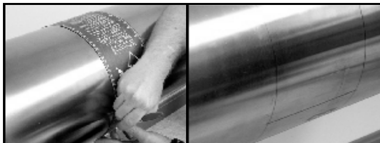
Figure 23: Marking the 3 o'Clock Position
